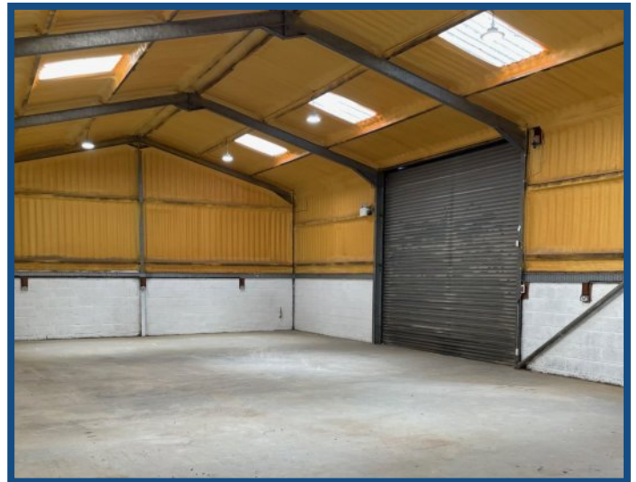
General Internal View of Workshop
